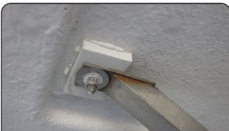
Photo 48: Support for "new" swim platform. Note some corrosion
