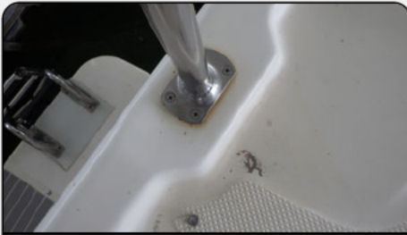
Photo 12: corrosion on the stanchion mounting.
